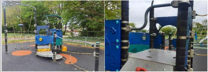
**Finding:** The unit is easily accessible and has an opening in **Action:** Monitor - No action given the risk assessment the barrier to steep play elements in excess of 500mm in contravention of BS EN 1176 Part 1
