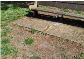
Finding: There are trip hazards at the edges of the surface Action: Remove trip hazard
