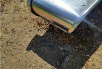
**Finding:** Hard fixing pins have been installed in the grass mat tiles within the impact area of the equipment. Grass mat pins should only be installed at the perimeter of the tiles, and outside of any equipment impact areas. NOTE - where grass mat wear pads have been provided and the impact area includes surrounding surfaces, the grass mats should be tucked into the turf, and not pinned
