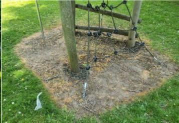
**Finding:** The grass mats are silted up and the soil is compacted; this may have an effect on the impact absorbing properties of the surface. Consideration should be given to HIC testing the surface to verify impact attenuating properties (https://playinspections.co.uk/inspectionservices/safety-surface-testing/)
