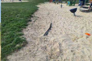
**Action:** Remove or resecure the exposed membrane and top up the surface to the correct level
