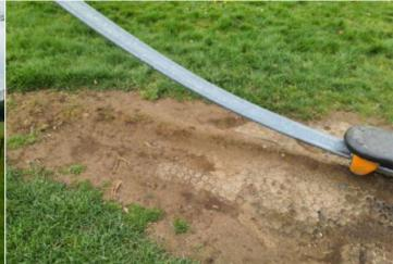
**Finding:** The grass mats are silted up, the soil is compacted **Action:** Reinstate as required and the area will become very slippery when the soil is wet.
