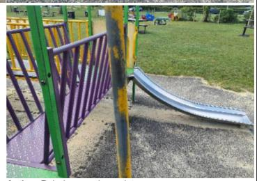
Finding: The paint has worn off the metalwork
