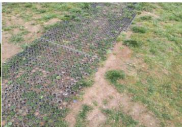
**Finding:** Fixing Pins have been installed in the impact areas **Action:** Remove pins from impact areas of the grass mats
