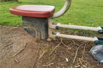
**Finding:** The distance between the underside of the item and the ground is less than the 60mm required by BS EN 16630
