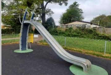
Finding: There is/are finger entrapment/s in the starting section of the slide and the item fails to meet the requirements of BS EN 1176 Part 1 4.2.7.6 Entrapment of fingers
