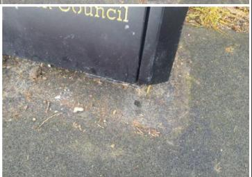
**Finding:** The bin is not securely fixed to the surface and there is some possibility of the item tipping or rolling over
