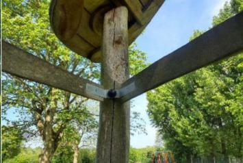
**Finding:** There are splits running through the timber that cross through or near fixing points and may cause instability in the future
