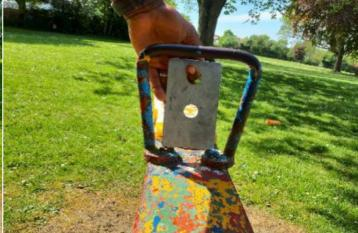
Finding: The item fails to meet the requirements of BS EN Action: Monitor - No action given the risk assessment 1176 Part 1 4.2.7.2 for head and neck entrapment in the handles
