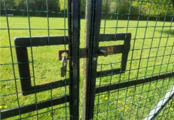
**Finding:** The maintenance gate was correctly padlocked at **Action:** Ensure that there are 12mm gaps throughout the the time of inspection, however this means that the inspector full range of motion on gate/s and between leaves where was unable to fully assess the gate relevant
