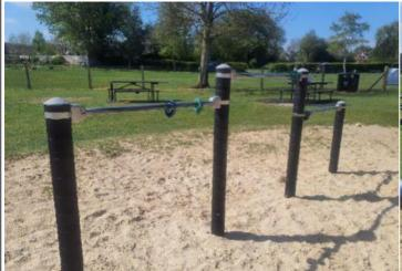
**Finding:** There is/are finger entrapment/s / crush in the Somersault bars fixing and the item fails to meet the requirements of BS EN 1176 Part 1 4.2.7.6 Entrapment of fingers
