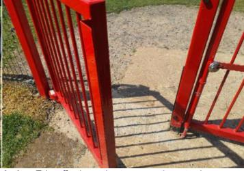
**Action:** Take effective action to ensure the gate closes between 4 and 8 seconds from 90 degrees
