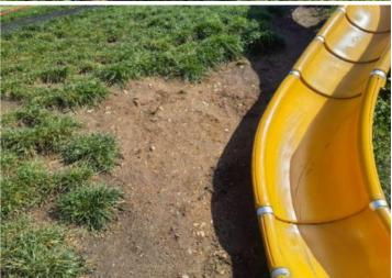
**Finding:** The grass has eroded within the impact area of the equipment and may not provide the necessary impact
