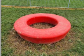
**Finding:** The bench/es is/are not securely fixed to the surface and there is some possibility of the item/s tipping or rolling over
