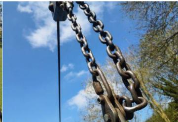
**Finding:** A secondary safety has been added and the chain **Action:** Replace worn chains links are worn excessively and require renewing.
