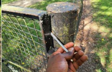
**Finding:** There are openings that are less than 12mm that could trap or crush fingers
