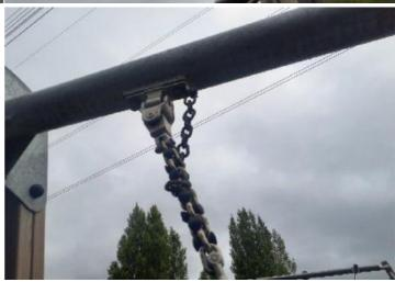
**Finding:** The secondary safety shackles are worn in excess **Action**: Replace worn shackles of 40% and require renewing
