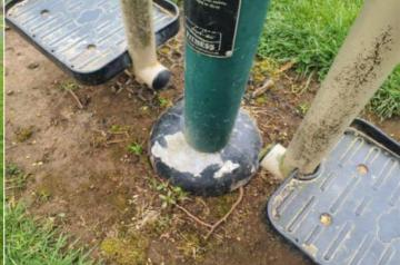
Finding: The paint is flaking off the metalwork
