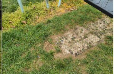
**Finding:** Fixing Pins have been installed in the impact areas **Action:** Remove pins from impact areas of the grass mats
