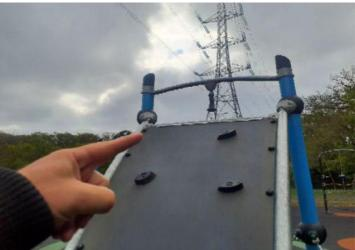
**Finding:** There is/are finger entrapment/s in the framework / **Action:** Monitor - No action given the risk assessment climbing wall and the item fails to meet the requirements of BS EN 1176 Part 1 4.2.7.6 Entrapment of fingers
