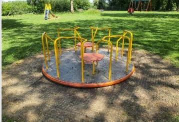
**Finding:** The distance between the underside of the roundabout platform and the playing surface is less than 60mm and contravenes the requirements of BS EN 1176 Part 5 which requires that the distance be maintained between 60mm-110mm for the entire circumference of the roundabout
