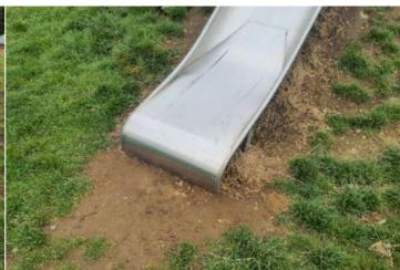
**Finding:** The grass has eroded within the impact area of the **Action:** Reinstate the grass or provide an all weather equipment and may not provide the necessary impact surface
