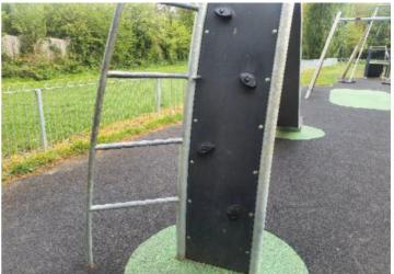
**Finding:** There is/are finger entrapment/s due to missing fixings and the item fails to meet the requirements of BS EN 1176 Part 1 4.2.7.6 Entrapment of fingers
