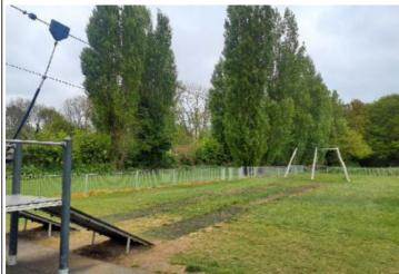
**Finding:** The edges of the grass mat surface are raised / lifting above the surrounding surface
