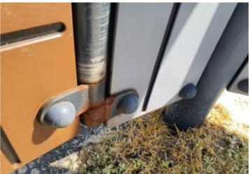
Finding: The paintwork on this item has been damaged or Action: Treat affected areas and repaint worn exposing the metal underneath which is rusting / corroding
