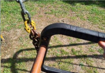
**Finding:** There are caps missing from the underside of the **Action:** Replace missing caps under the seats seats
