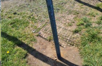
**Finding:** The edges of the grass mat surface are raised / lifting above the surrounding surface
