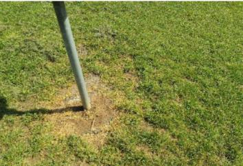
**Finding:** There is moderate damage to the grass matrix tile **Action:** Repair the damaged areas of surfacing surface
