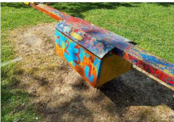
Finding: There is no gaiter protection for accessible moving Action: Monitor - No action given the risk assessment parts (possible shear trap) as recommended in BS EN 1176
