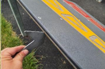
Finding: The item has exposed edges and corners that are Action: Provide a 3mm radius to all exposed edges and sharp, or with a radius of less than 3mm, and does not meet corners, or remove sharp edge the requirements of BS EN 1176 Part 1 - 4.2.5
