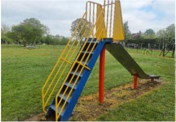
Finding: The paintwork on this item has been damaged or Action: Treat affected areas and repaint
