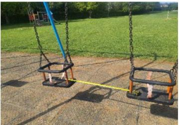
**Finding:** The seats are too close to each other as defined in **Action:** Monitor - No action given the risk assessment BS EN 1176 Part 2; this is a low risk failure and no remedial action is required
