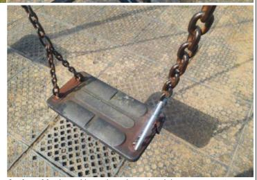
**Finding:** The chain openings are in excess of 8.6mm and do not meet the recommendations of BS EN 1176 Part 1
