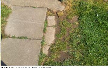
Finding: There are trip hazards at the edges of the surface Action: Remove trip hazard
