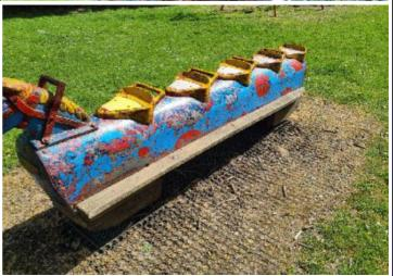
**Finding:** There is no gaiter protection for accessible moving **Action:** Monitor - No action given the risk assessment parts (possible shear trap) as recommended in BS EN 1176 Part 1; 4.2.6 Moving Parts
