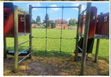
**Finding:** The grass mats are silted up and the soil is compacted; this may have an effect on the impact absorbing properties of the surface. Consideration should be given to HIC testing the surface to verify impact attenuating properties ( https://playinspections.co.uk/inspectionservices/safety-surface-testing/)
