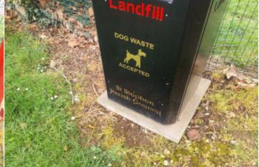
**Finding:** The bin is not securely fixed to the surface and there is some possibility of the item tipping or rolling over
