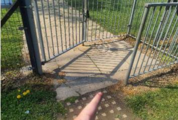
Finding: There are trip hazards at the edges of the surface Action: Remove trip hazard
