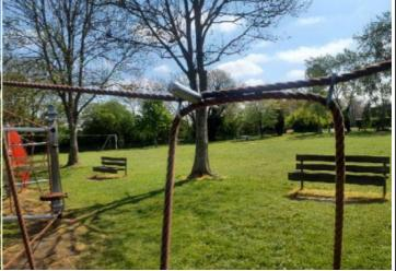
**Finding:** There is/are finger entrapment/s in the rope connection and the item fails to meet the requirements of BS EN 1176 Part 1 4.2.7.6 Entrapment of fingers
