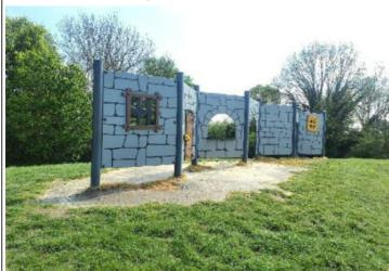
**Finding:** There is a potential crush point between the play panel door in contravention of BS EN 1176 Part 1 - 4.2.7.6 gaps whose dimensions change during use of the equipment shall have a minimum dimension in any position of 12mm
