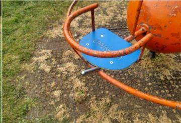
**Finding:** There is/are finger entrapment/s in the framework / **Action:** Monitor - No action given the risk assessment seat and the item fails to meet the requirements of BS EN 1176 Part 1 4.2.7.6 Entrapment of fingers
