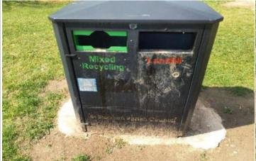
**Finding:** The surface has eroded and the foundations are exposed
