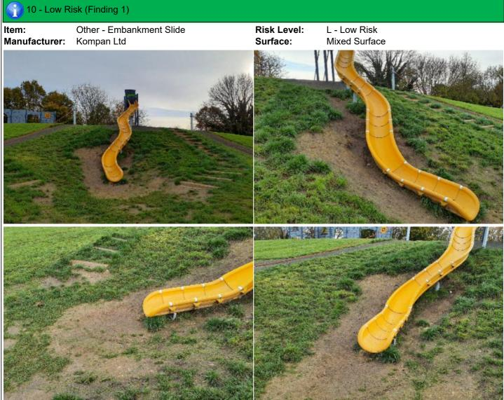
**Finding:** The grass has eroded within the impact area of the **Action:** Reinstate the grass or provide an all weather equipment and may not provide the necessary impact attenuating properties for the equipment fall height; the surface may also be slippery in wet weather
