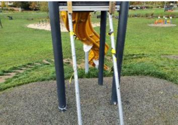
**Finding:** NOTE - The item has been isolated from use due to accidents that have occurred. The access element has been removed and a full inspection could not be undertaken of the platform / starting area
