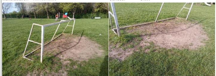
Finding: The surface has eroded in some areas and may be Action: Reinstate the surface slippery in wet conditions
