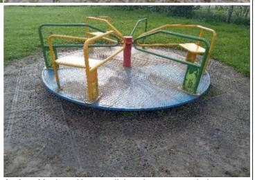
**Finding:** The distance between the underside of the roundabout platform and the playing surface is in excess of 110mm and contravenes the requirements of BS EN 1176 Part 5 which requires that the distance be maintained between 60mm-110mm - for the entire circumference of the roundabout
