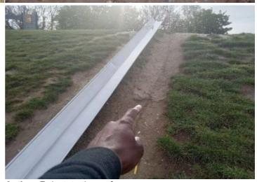
**Finding:** The concrete foundation forms a projecting obstacle / hard object within the free space of the equipment, in contravention of the requirements of BS EN 1176 Part 1
