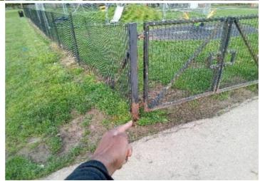
**Finding:** Parts of the steel on this item have corroded excessively and the metal has perforated in places
