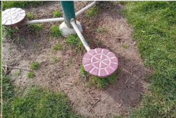
**Finding:** The deflection of the rotating user station exceeds **Action:** Monitor - No remedial work recommended the maximum 105 degrees required by BS EN 16630
