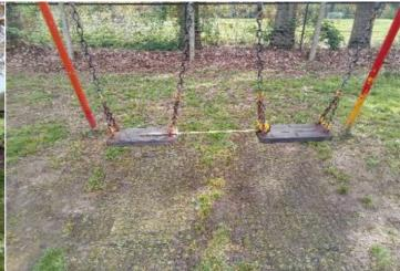
Finding: The seats are too close to each other as defined in Action: Monitor - No remedial work recommended BS EN 1176 Part 2; this is a low risk failure and no remedial
