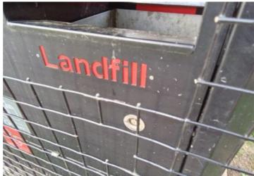
**Finding:** The fence panel has been cut to allow access to the litter bin from the outside of the play area. The cut sections have projections and sharp edges
