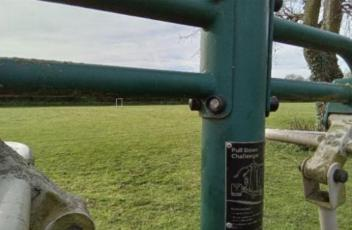
**Finding:** There is/are bolt cap covers missing or damaged on the item
