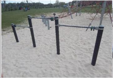
**Finding:** There is/are finger entrapment/s / crush in the Somersault bars fixing and the item fails to meet the requirements of BS EN 1176 Part 1 4.2.7.6 Entrapment of fingers
