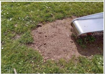
**Finding:** The grass mats are silted up, the soil is compacted **Action:** Reinstate as required and the area will become very slippery when the soil is wet.
