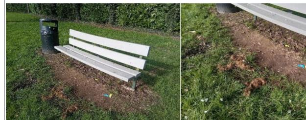
**Finding:** The surface has eroded in some areas and may be **Action:** Reinstate the surface slippery in wet conditions
