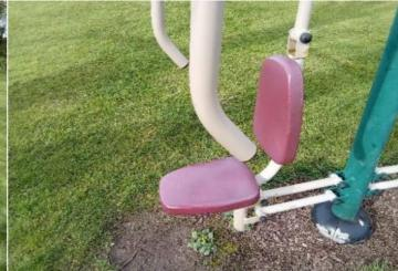
Finding: One or more handgrip(s) are damaged or missing. Action: Replace missing or damaged handgrips
