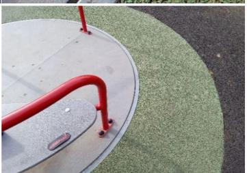
**Finding:** Roundabout is snagging against outer edge causing difficulty in rotating
