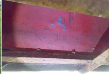
**Finding:** There is no gaiter protection for accessible moving **Action:** Monitor - No remedial work recommended parts (possible shear trap) as recommended in BS EN 1176
