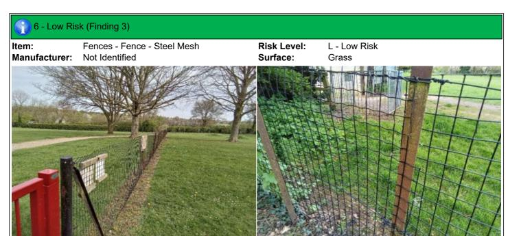
Finding: The paintwork on this item has been damaged or Action: Treat affected areas and repaint worn exposing the metal underneath which is rusting / corroding
