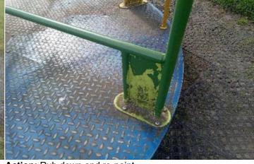
Finding: The paint is flaking off the metalwork
