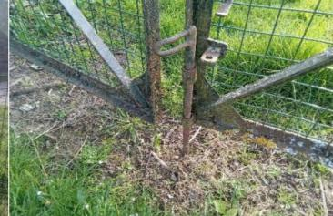
Finding: The gate has no drop bolt sleeves and/or drop bolts fitted
