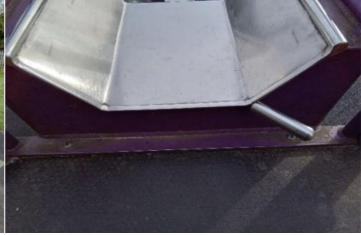
**Finding:** There is/are finger entrapment/s in the slide platform and the item fails to meet the requirements of BS EN 1176 Part 1 4.2.7.6 Entrapment of fingers
