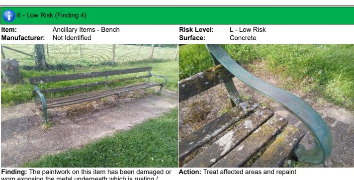
worn exposing the metal underneath which is rusting / corroding
