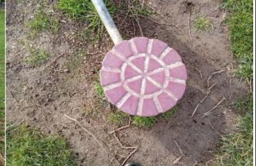
**Finding:** The rotating user station is not appropriately marked with a guideline of user direction and/or the original position as required by BS EN 16630
