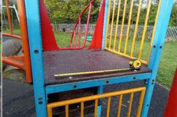
Finding: There is an opening in the barriers exceeding the Action: Monitor - No remedial work recommended width allowed (500mm) in BS EN 1176, this is a low risk failure and no remedial action is required
