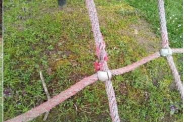
Finding: The rope has worn and wire strands are exposed
