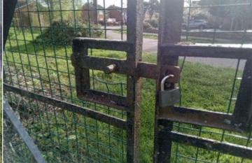
**Finding:** The maintenance gate was correctly padlocked at **Action:** Ensure that there are 12mm gaps throughout the the time of inspection, however this means that the inspector full range of motion on gate/s and between leaves where was unable to fully assess the gate relevant
