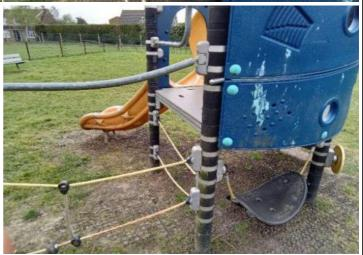
Finding: There is/are finger entrapment/s in the barrier next Action: Monitor - No remedial work recommended to access element and the item fails to meet the requirements of BS EN 1176 Part 1 4.2.7.6 Entrapment of fingers
