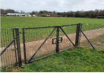
**Finding:** The area under the gate has eroded leaving uneven areas, or the concrete foundations exposed, resulting in trip hazards at the entrance/exit to the playground
