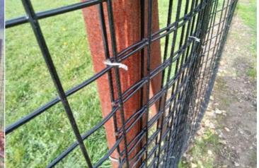
Finding: Cable ties have been used on the item and there are sharp projecting ends
