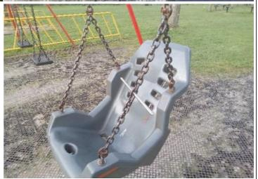
**Finding:** The chain openings are in excess of the 8.6mm as **Action:** Monitor - No remedial work recommended recommended by BS EN 1176
