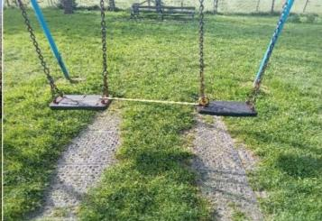
Finding: The seats are too close to each other as defined in Action: Monitor - No remedial work recommended BS EN 1176 Part 2; this is a low risk failure and no remedial action is required
