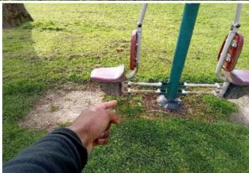
**Finding:** The distance between the underside of the item and the ground is less than the 60mm required by BS EN 16630
