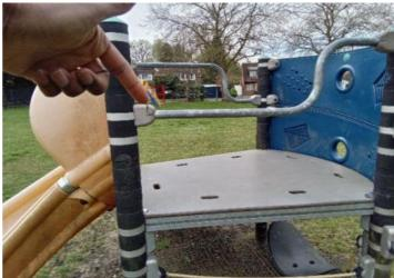
**Finding:** A number of fixing(s) have worked loose on guardrail
