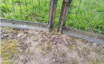
Finding: The gate has no drop bolt sleeves and/or drop
