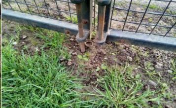
**Finding:** The gate has no drop bolt sleeves and/or drop bolts fitted
