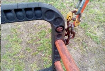
Finding: There are caps missing from the underside of the Action: Replace missing caps under the seats
