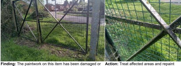
worn exposing the metal underneath which is rusting / corroding
