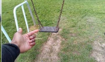
Finding: The swing seat connectors are loose Action: Tighten to secure
